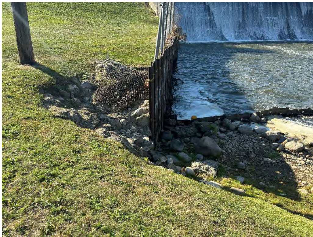
Photo 16 – Erosion at Downstream End of East Abutment - Monitor
