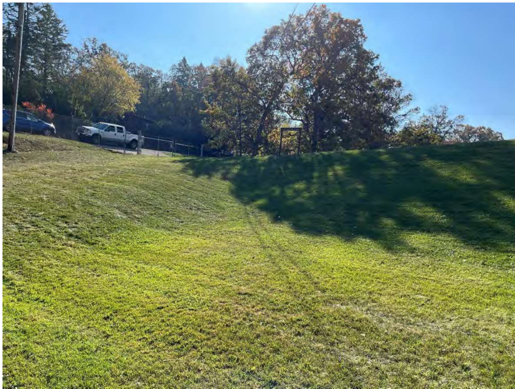
Photo 6: Downstream Face of East Embankment
