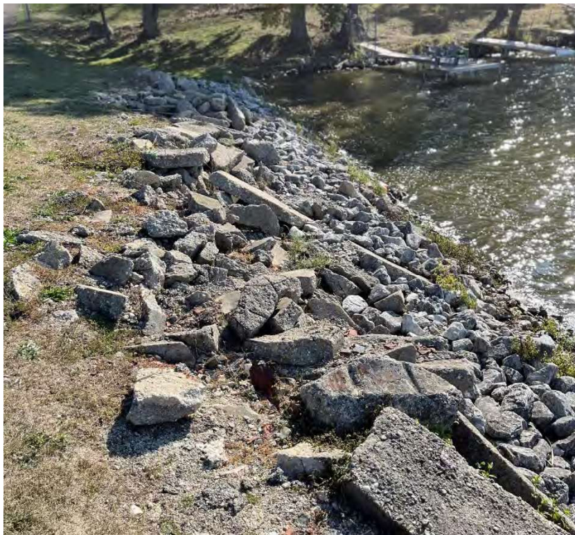
Photo 12: East Embankment – Upstream Face Riprap (Facing East)
