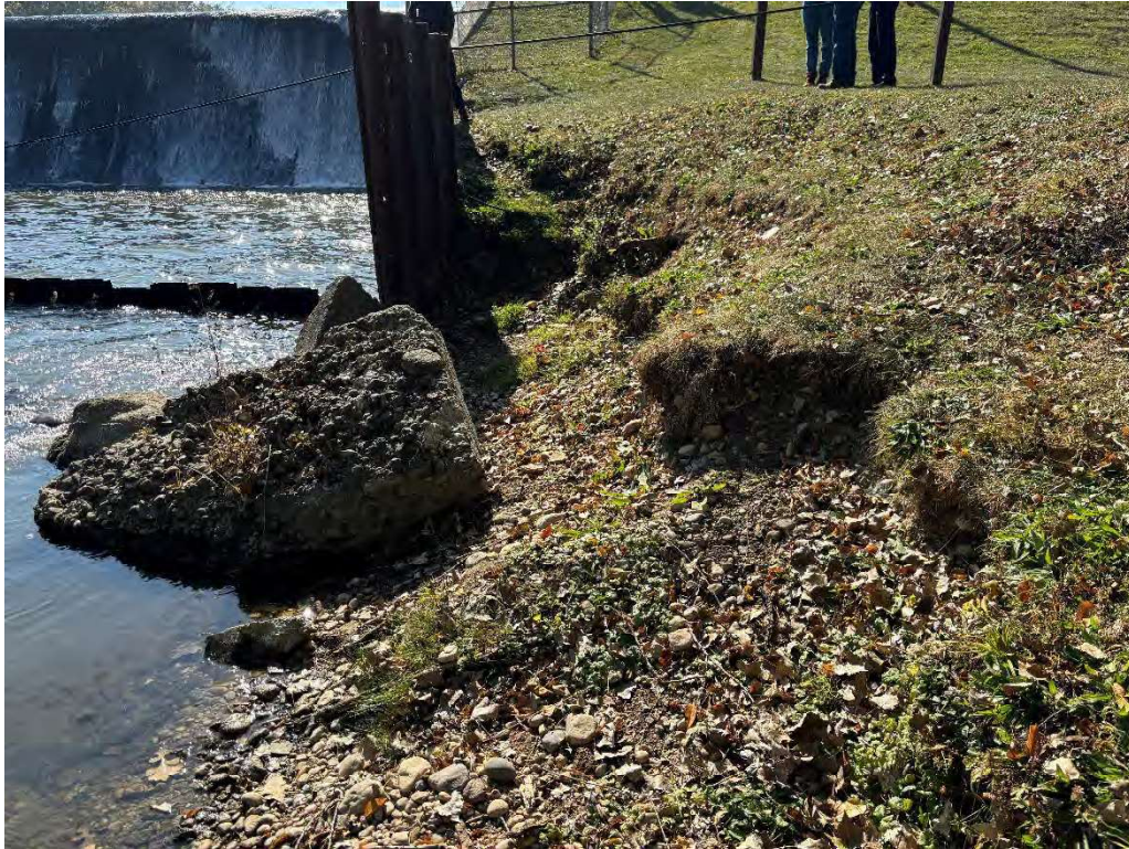
Photo 17 - Erosion at Downstream End of East Abutment - Monitor
