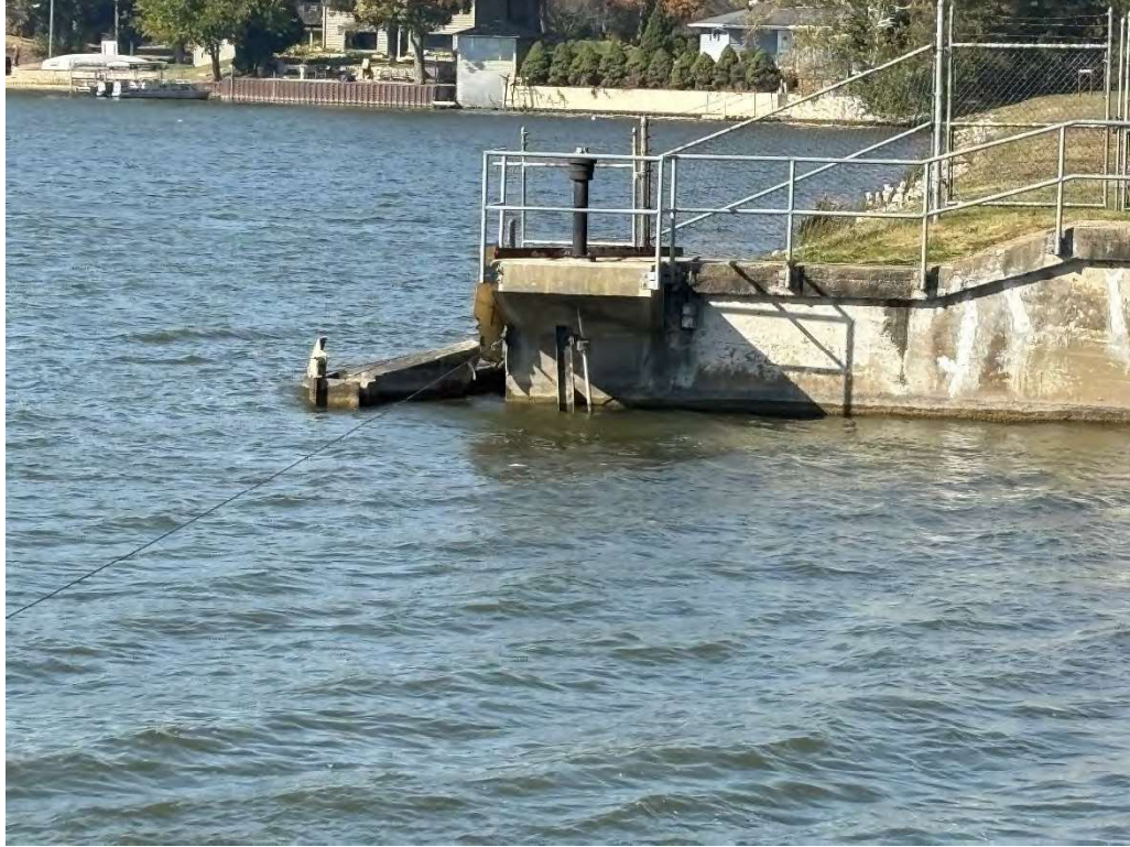
Photo 9: West Sluice Gate – Shaft and steel protection framing is bent – Gate is inoperable
