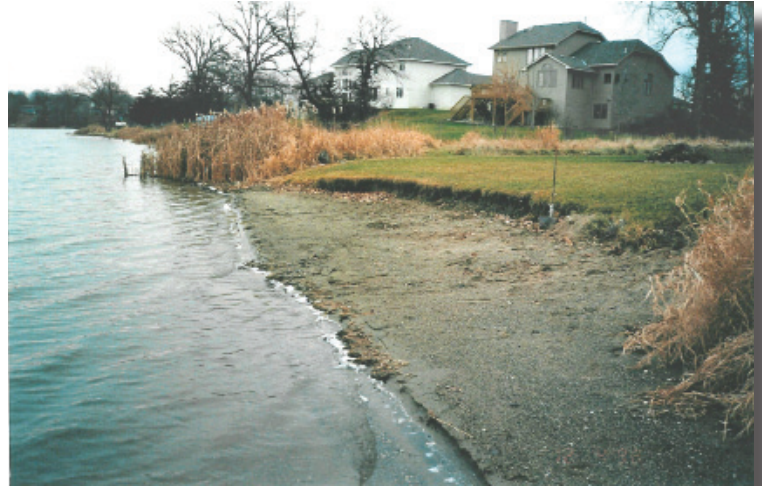
Contrast the eroded shoreline lacking vegetation (foreground) with the well-vegetated, uneroded shoreline in the distance.
