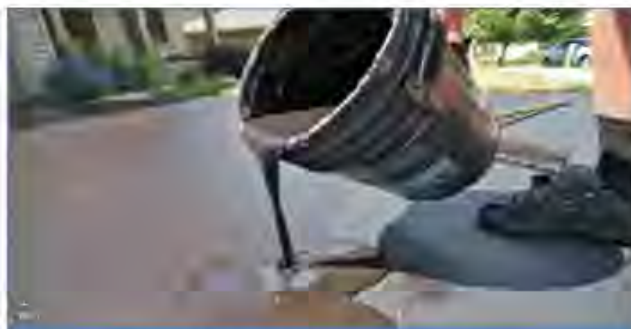
Pouring seal coating on a driveway. photo: Minnesota Pollution Control Agency
